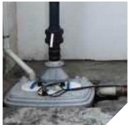
-1. kat zeminine kurulan Sanicubic 2 XL
